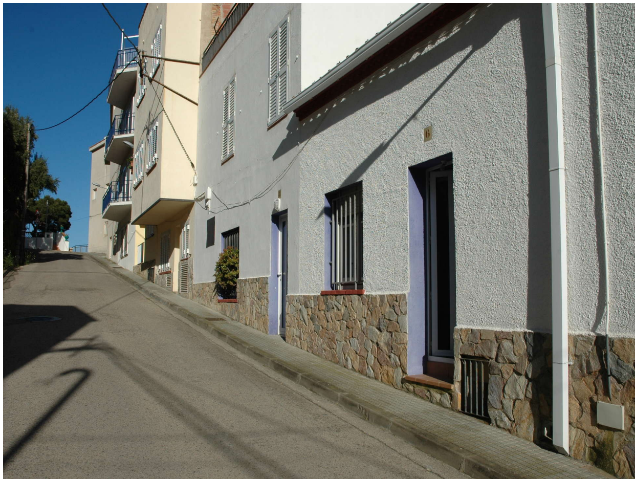
Ground floor in a village house near the beach
